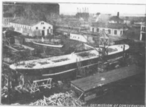
REINFORCED CONCRETE BOAT S.S. Conerita, prior to LAUNCHING AT MONTREAL.
