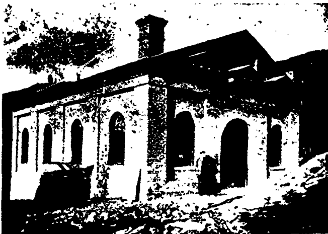
FIG. 1.—THE SUB-STATION AT ROSSLAND.
