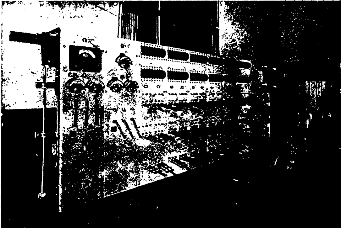
MONTREAL COTTON COMPANY'S PLANT—GENERATOR AND FEEDER PANELS.
