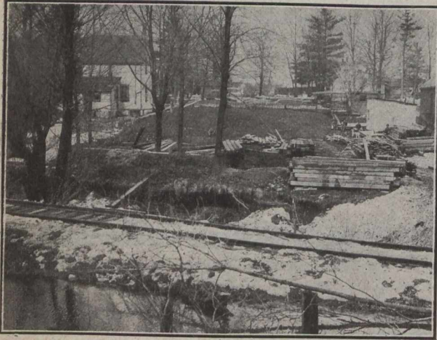
Fig. No. 5.—Bridge Site at Start of Work
