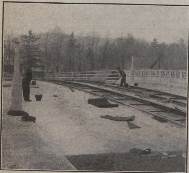
Fig. No. 11.—Waterproofing the Roadway and Track Allowance
