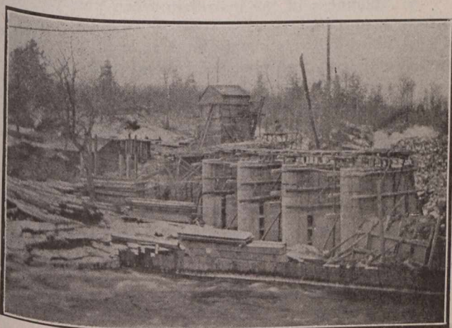
Fig. 4.—Erection of Power Plant, Piers Completed.
