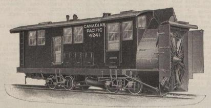
Rotary Snow Plows have been in successful operation under the most trying conditions for over twenty-five years. They keep the road open. Work with certainty and regularity. Do not spread the rails. Do not derail. Heavy snowstorms and deep drifts increase operating expenses.
