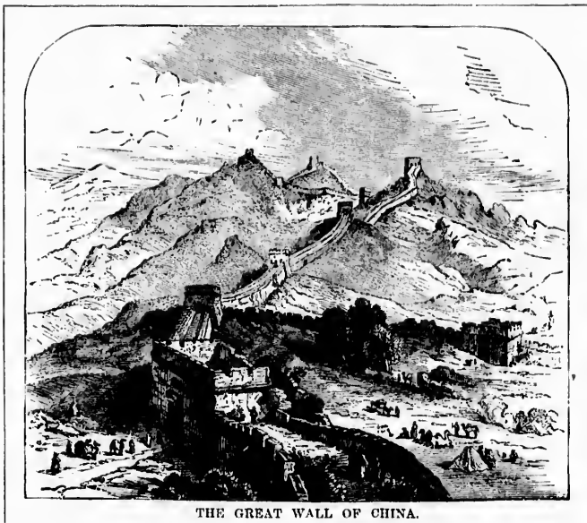
THE GREAT WALL OF CHINA.
