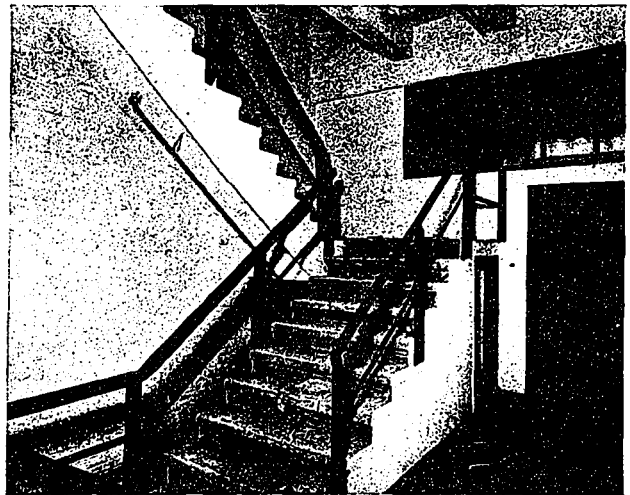
Fig. 10—VIEW OF FIREPROOF STAIRWAY, OGILVIE BUILDING, TORONTO, SHOWING THE SOLID CONCRETE TREADS AND IRON HANDRAIL. IN THE BACKGROUND TO THE RIGHT MAY BE SEEN ONE OF THE WALLS ENCLOSING THE PASSENGER ELEVATOR SHAFT. THE WINDOW SHOWN HAS METAL SASH AND FRAME, AND IS GLAZED WITH WIRED GLASS.
