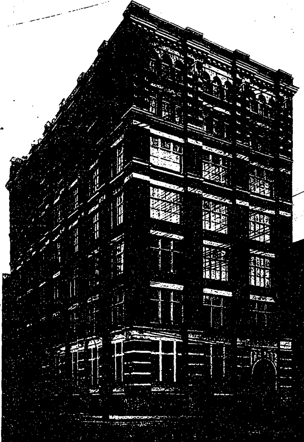
Fig. 8—WAREHOUSE AND OFFICE BUILDING RECENTLY ERECTED BY THOMAS OGILVIE & SONS, AT TORONTO. THIS STRUCTURE IS AN EXCELLENT ILLUSTRATION OF STEEL FRAME ENCASED WITH CONCRETE ON EXPANDED METAL LATH, A TYPE OF CONSTRUCTION BECOMING QUITE POPULAR, AND ONE WELL ADAPTED FOR WAREHOUSES. NO EFFORT OR EXPENSE HAS BEEN SPARED IN PLAN, ARRANGEMENT, SELECTION OF MATERIALS, OR APPLIANCES TO RENDER THIS BUILDING AS THOROUGHLY FIREPROOF AS MODERN BUILDING SCIENCE WILL PERMIT OF. BURKE & HORWOOD, ARCHITECTS, TORONTO. EXPANDED METAL AND FIREPROOFING CO., CONSULTING ENGINEERS.
