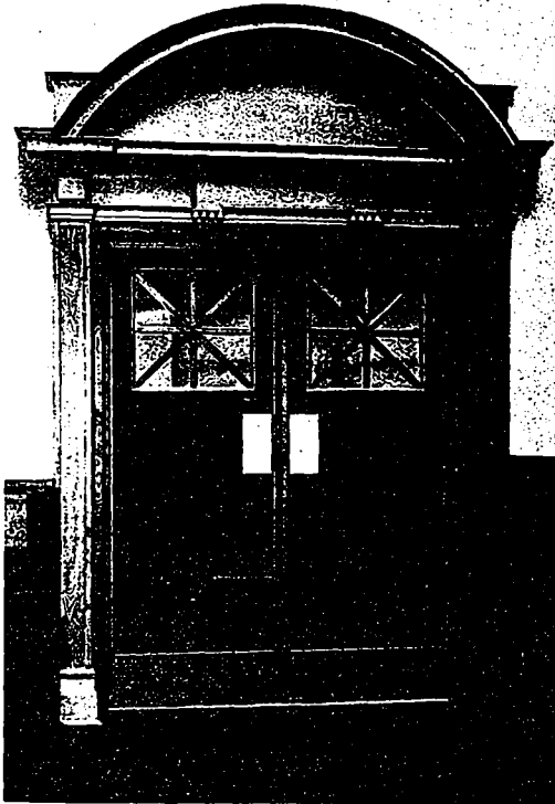
DETAIL OF CLOTH COVERED DOOR, LEADING FROM STAGE FRONT TO FOYER. DARLING & PEARSON, ARCHITECTS.
