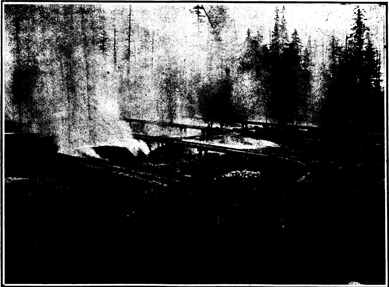
Roast Yard at Tye Copper Co's smelter, showing Permanent Trestles and Burning Ore Piles.
