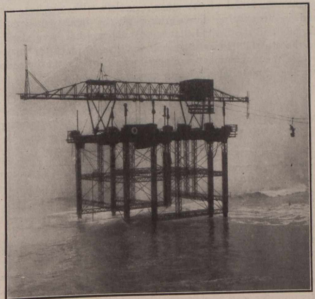
Men may be conveyed in baskets to the stage in rough weather.
