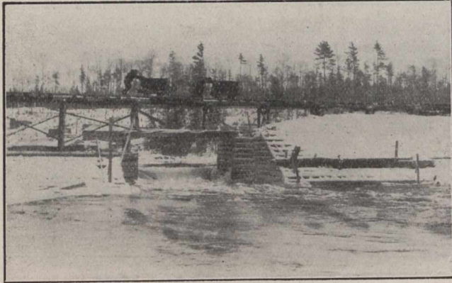
Showing timber dam north side.
