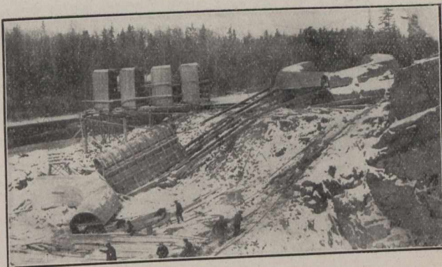
Showing forms for power house.
