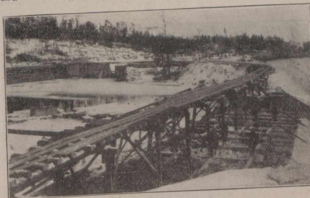
Timber dam and canal intake.
