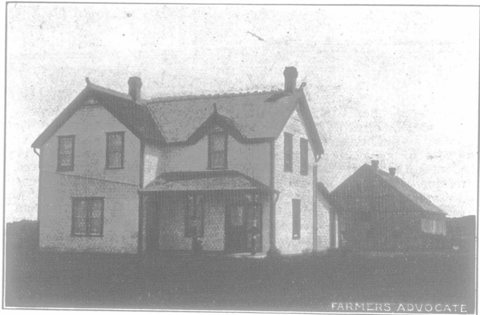
PERCY SWITZER'S FARM BUILDINGS NEAR LACOMBE, ALTA.
