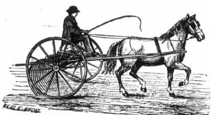
The head is so attached that it permits the teeth to accommodate themselves to uneven ground, the wheels running upon an elevation will not raise the teeth from the ground. By the raising attachment the operator can throw the teeth of the rake higher in passing over the winrow than any other manufectured.
