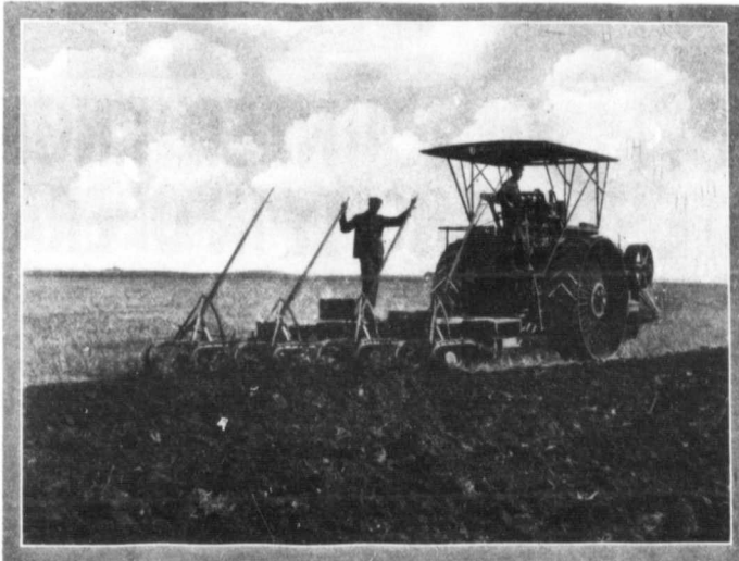
A Buffalo Pitts Gas Tractor pulling an 8-bottom John Deere Engine Gang
