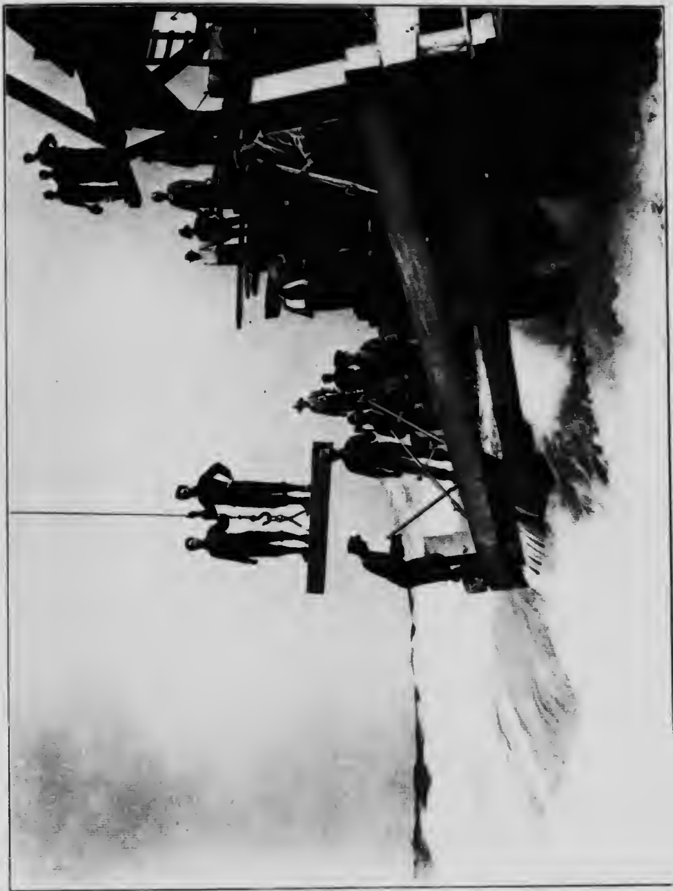
Photograph showing Cascade and launching of a crib. It was at this point that the only fatal accident during construction of the crib occurred; one of the workmen who fell into the river being carried over the falls.
