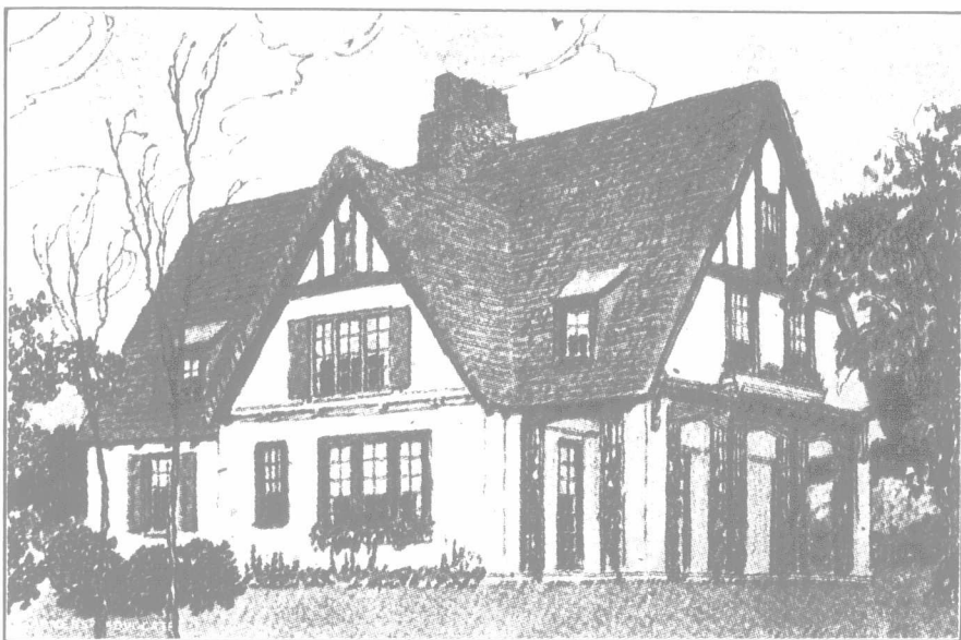
Grouped Windows and Long Roof Lines.
