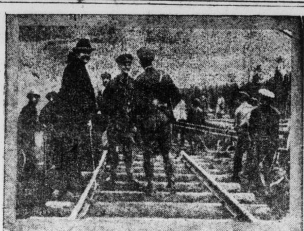
In the Far North—Canadian and American railway men replacing a piece of track and a bridge south of Archangel, Russia, which had been destroyed by the Bolsheviks.
