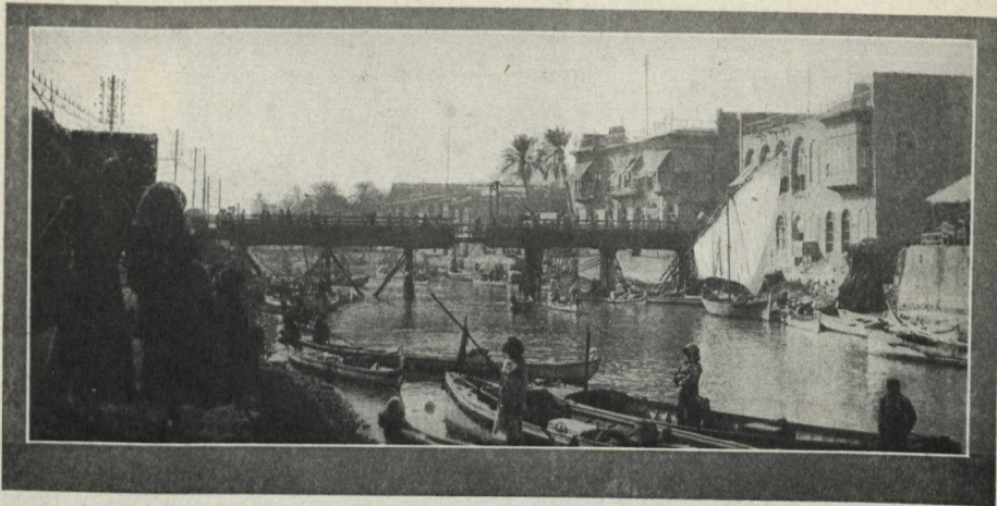
Whiteley Bridge, Ashar Creek, Basrah
