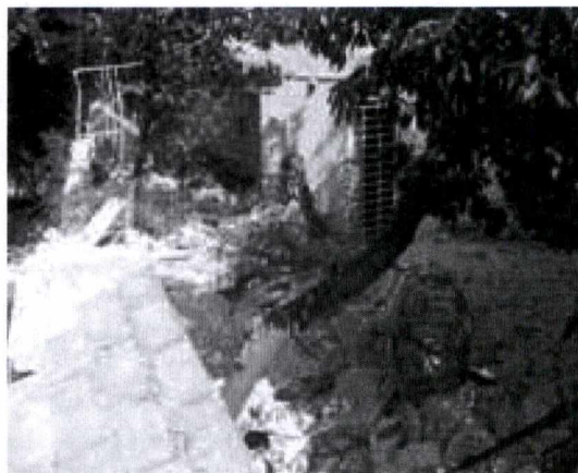
Haiti: employee residence, damaged by the earthquake
