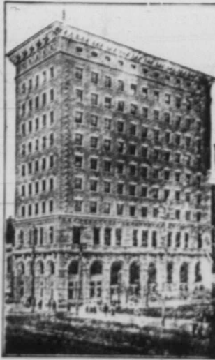
Union Bank Building, Winnipeg
