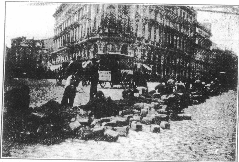
Laying Callender Mains at MARDID.
