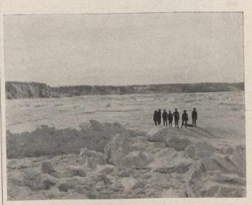
Fig 1.—Showing a cut in the Cap Rouge ice bridge in March, 1909. This is pack ice with frazil underneath. Photo taken from the "Montcalm."
