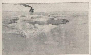
Fig. 9.—C.C.S. ''Lady Crey'' backed down the channel ready to come forward full speed into the ice. The V groove of the ship's prow may be seen in the foreground. The smoke of the ''Montcalm'' may be seen on the horizon.
