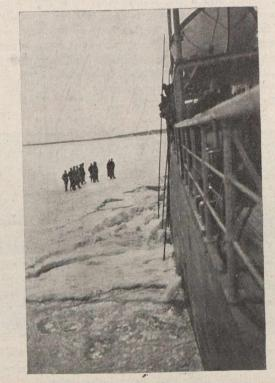
Fig. 6.- The "Montcalm" stuck for 10 hours in the ice below the Richelieu Rapids. Observe the effect of the circulating water in removing the frazil.
