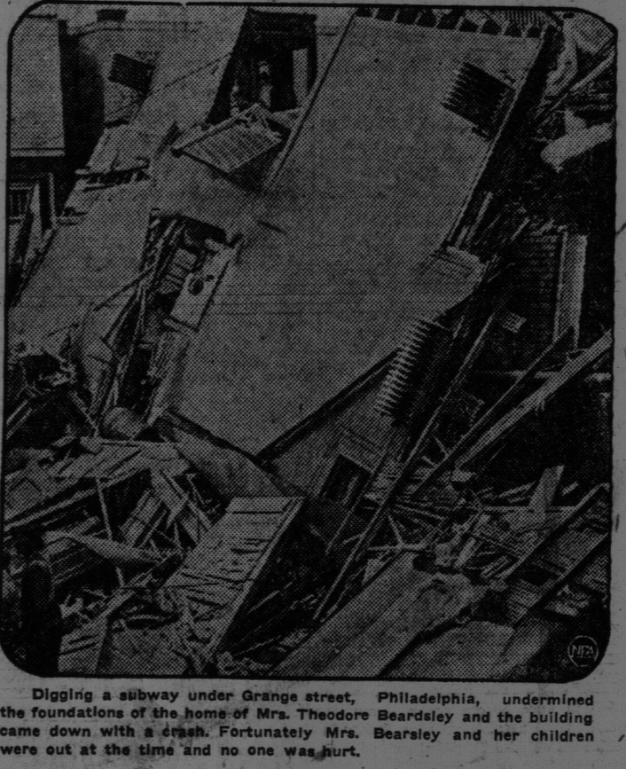
Digging a subway under Grange street, Philadelphia, undermined the foundations of the home of Mrs. Theodore Bearseley and the building came down with a crash. Fortunately Mrs. Bearseley and her children were out at the time and no one was hurt.
