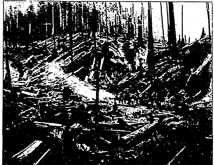
GENERAL VIEW OF LOGGING OPERATIONS.
