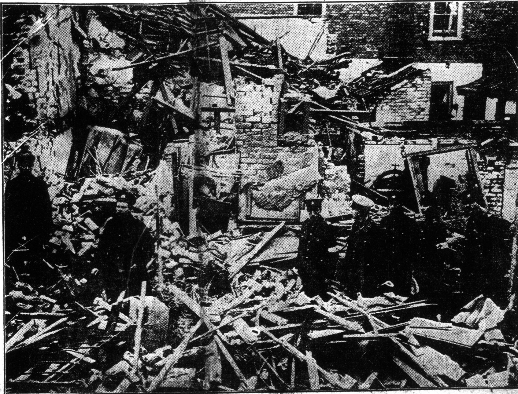
General view of two houses in Bentinck street, King's Lynn, after the bombardment by German air raiders.
