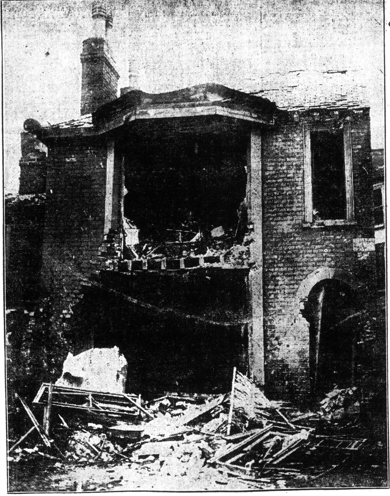
DAMAGE DONE TO A HOUSE IN ST. PETER'S PLAIN, YARMOUTH
