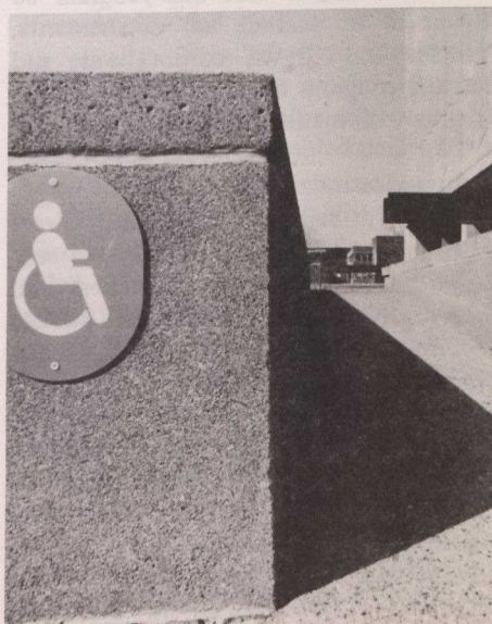
Ramps for building accessibility.
