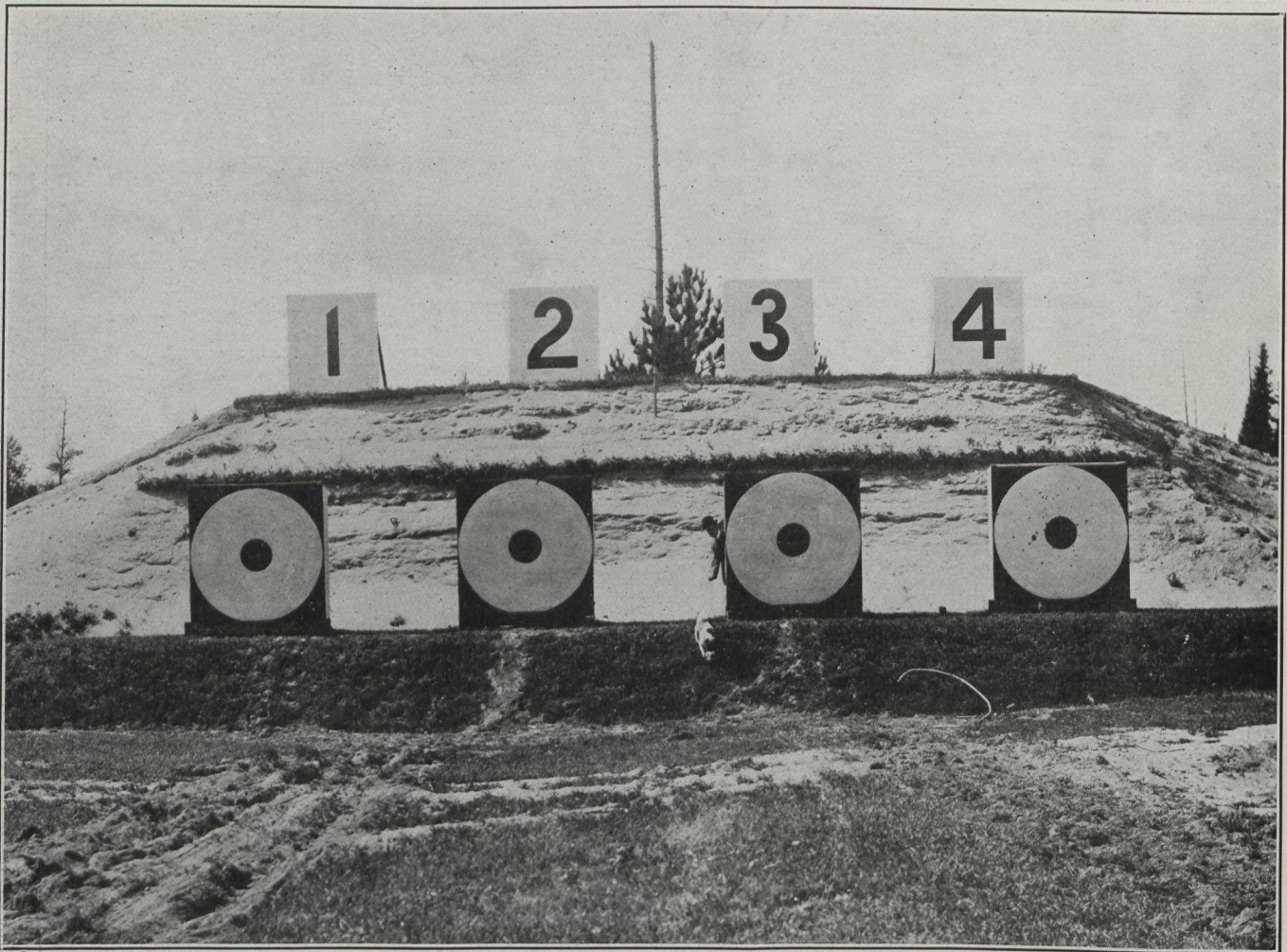
At Camp Petawawa The Peters target, which is installed at Petawawa, Ontario, is an invention of the late Lt.-Col. Peters. This target is designed to do away with markers. It is of delicate construction and the telegraphic system is utilized. The target was first installed at Long Branch, Ont., where the butts of the Toronto regiments are located. It was proven satisfactory, and some years ago Col. Peters demonstrated the target at the Dominion Rifle Association Meet at Ottawa.
