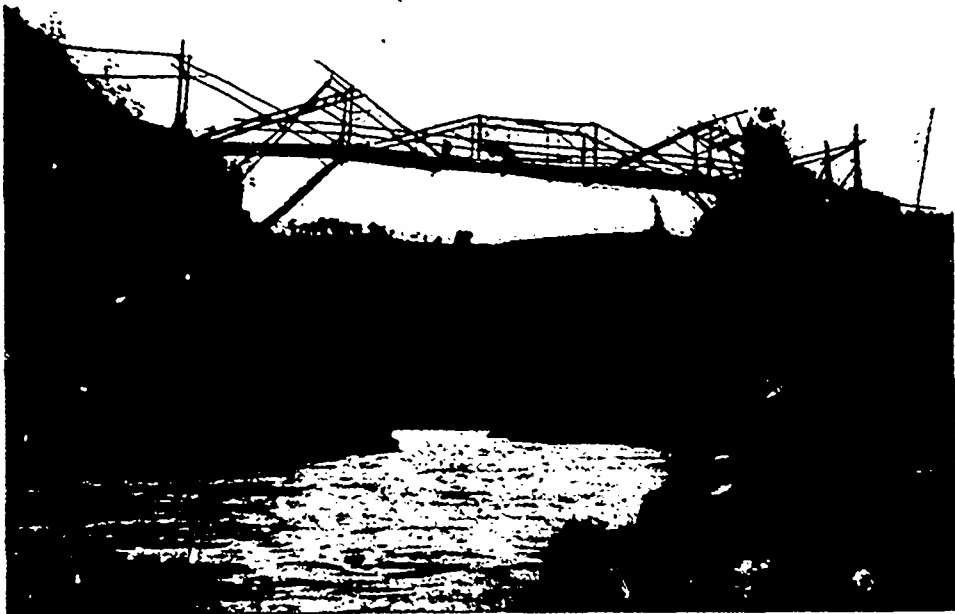
Bridge across Bulkley River at Ahwillgate: constructed by Indians of round poles and telegraph wire.
