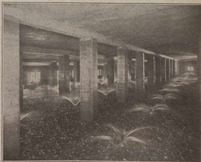
FILTER IN OPERATION
