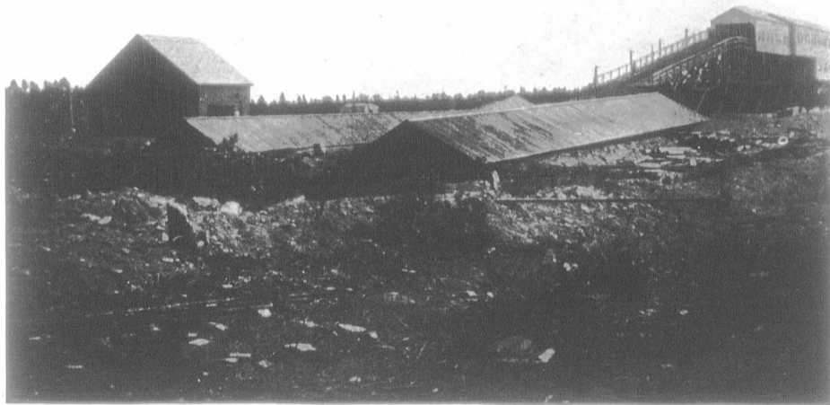
Mouths of Slopes. Compressor House and Bankhead, Dominion No. 21 Colliery
