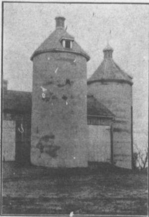
Two of the Four Silos at Prospect Farm. The silo in the background is 18 by 26 feet. The other three silos are smaller. Altogether they hold the corn from 60 acres.
