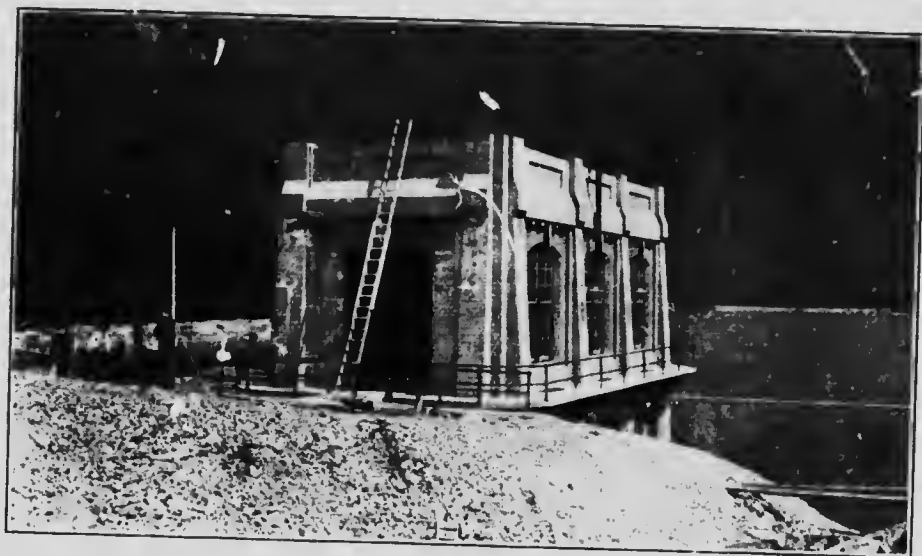
Power Plant No. 2.—Intake at Lake Buntzen.
