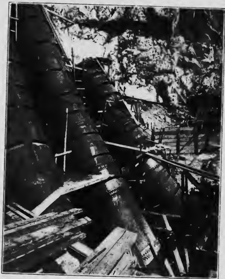
Plant No. 2, Lake Buntzen.—View showing three pipe lines at entrance to line tunnels behind Power House No. 2.
