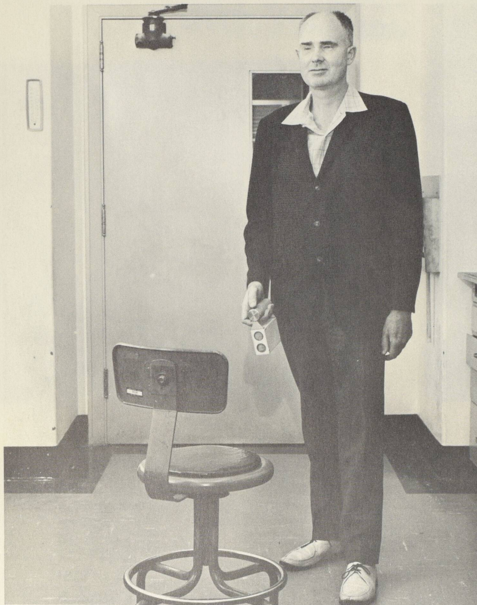
James Swail demonstrates his ultrasonic obstacle detector in office corridor.
