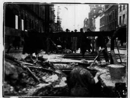
DRILLING UNDERGROUND CHANNELS UNDER DIFFICULTIES. On account of the heavy rains the work of excavating under Yongeet and Adelaide-street has been badly hampered, the workmen of neces-having to go slowly for fear of cave-ins.
