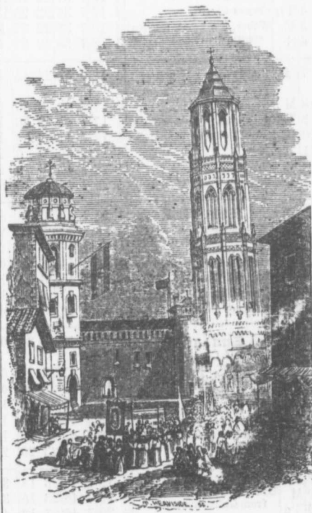
LEANING TOWER, SARAGOSSA.
