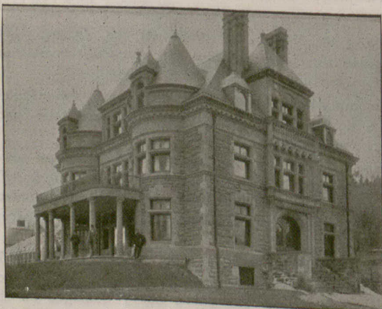
Residence of Jas. Ross, Montreal—Built of Miramichi Sandstone.
