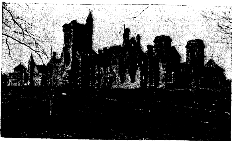
THE MAIN BUILDING AFTER THE FIRE.
