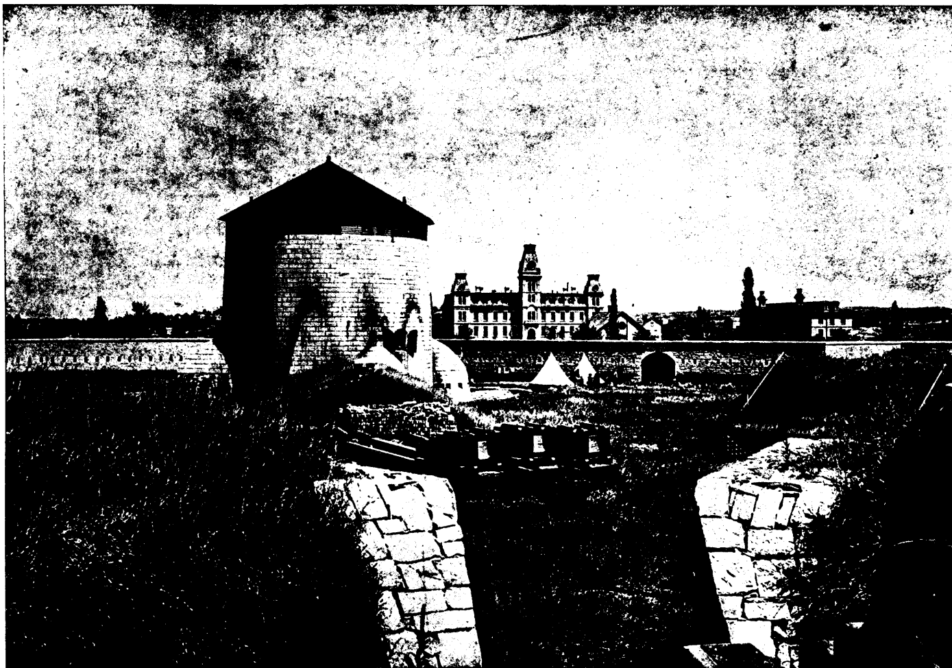
3 MARTELLO TOWER AT FORT FREDERIC, NEAR KINGSTON, DAMAGED BY FIRE. 14th MAY.
