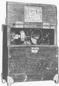
FIG. 3—PORTABLE TRAIN TELEPHONE SET
