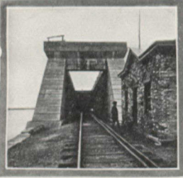
Victoria Tubular Bridge, showing construction of present Bridge.
