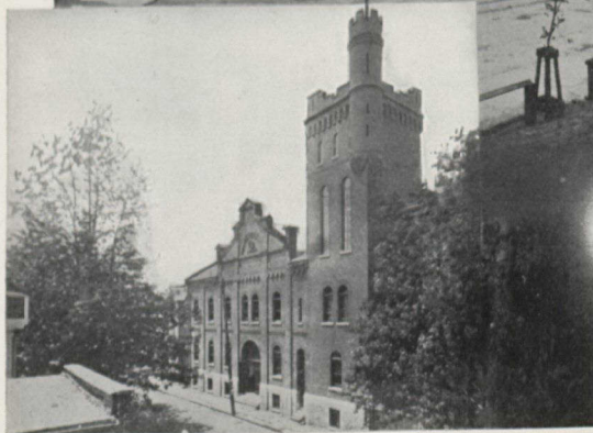
Drill-Hall and Victoria Rifles' Armoury.
