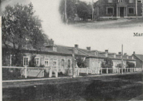
Cottages at Valleyfield.
