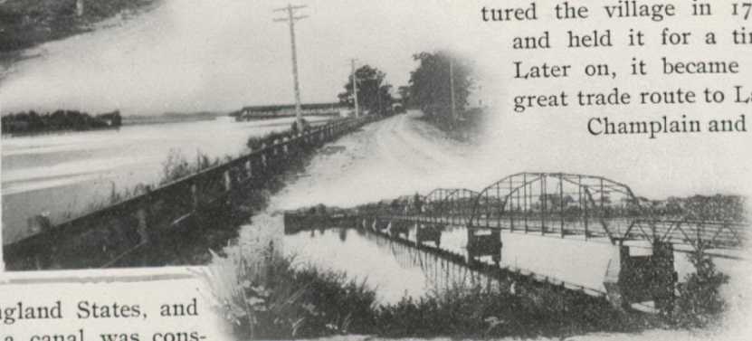
The Highway Bridge.
