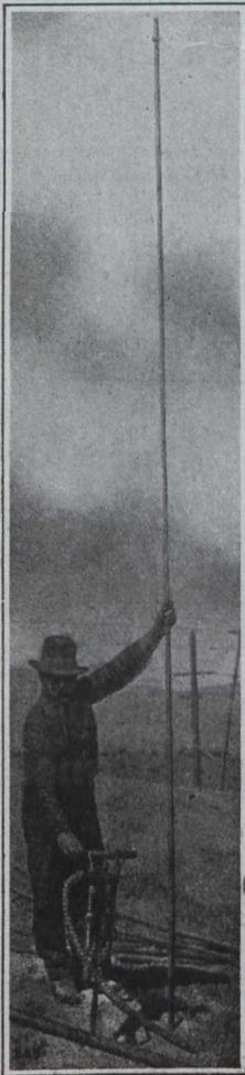
Waugh "Clipper" drilling with 22 ft. steels in the ballast pit of the C. M. & St. P. Ry., Co., at Vendome, Mont.
