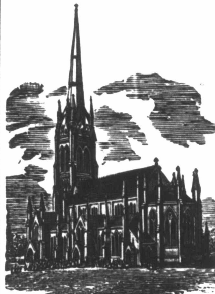
St. James' Cathedral, King St., Toronto, contains 500,000 cubic feet of space and is successfully heated with four of our Economy Heaters.
