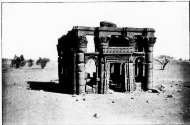
Naga—Roman Building in the Desert (Showing the Transition from Egyptian to Roman Style)
