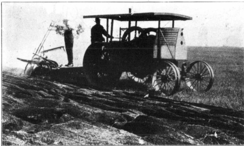
15 H.P. Gas Tractor Pulling a 2-Bottom 14-Inch Cliver Engine Gang.
