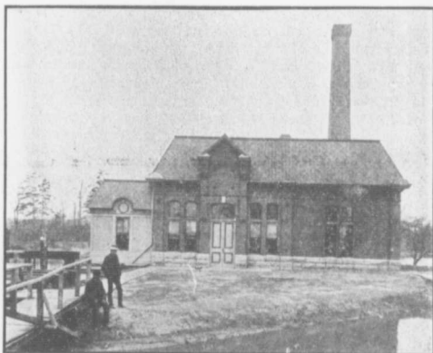
WATERWORKS PUMPING STATION
