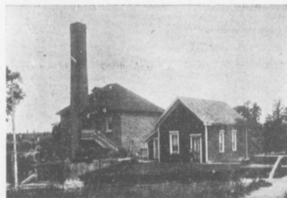
ELECTRIC LIGHT STATION.
