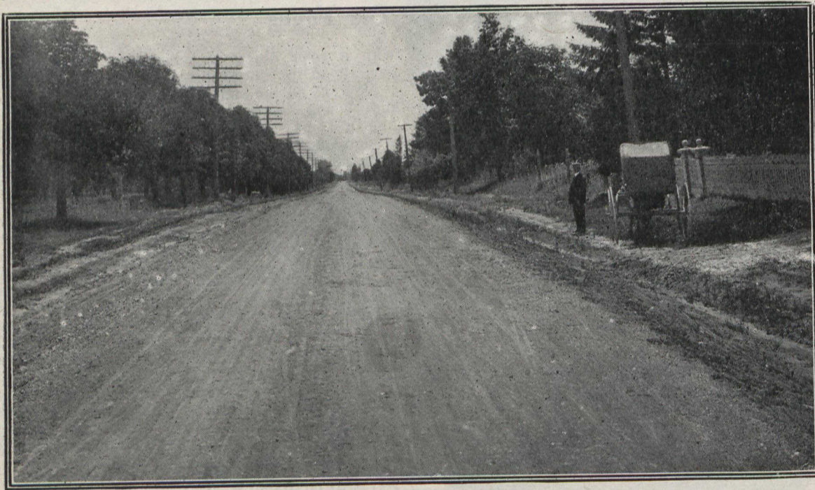
Solving the Problem. Dundas Street, Near Toronto—a Macadam Road 3¼ Miles in Length, Built by Mr. J. C. Eaton, and Hence Known as the Eaton Road.
