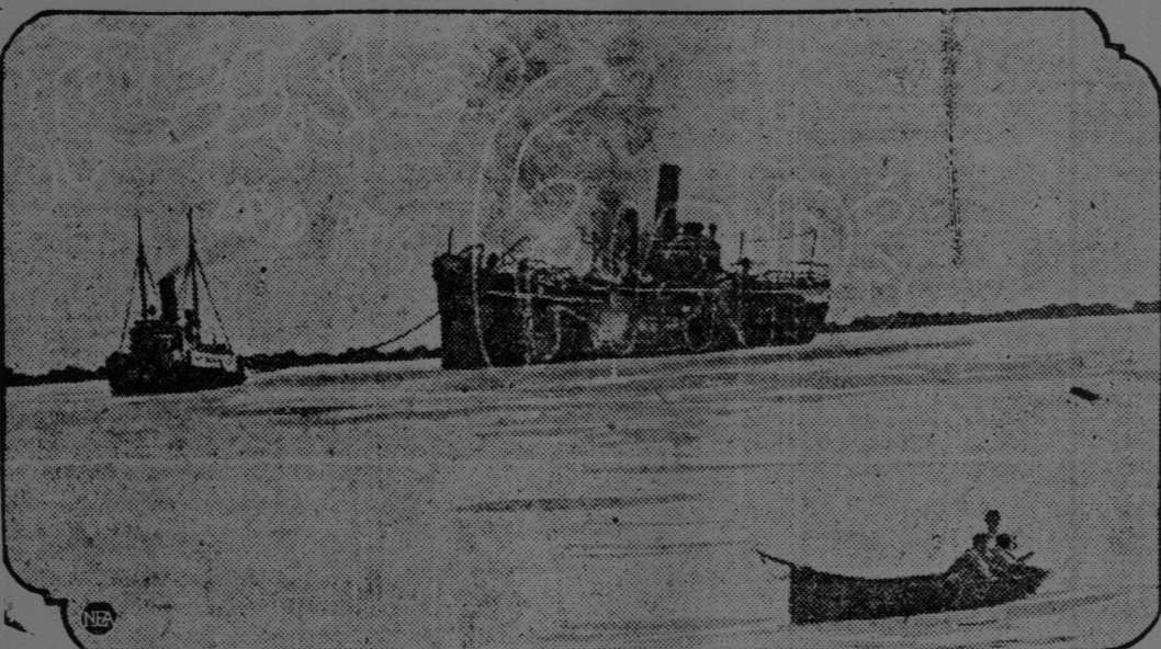
The burning steamship Comanche being towed up the St. John's river into Jacksonville, Fla. This shows the vessel still smouldering, nothing but the shell remaining after the fire had swept through the ship.
