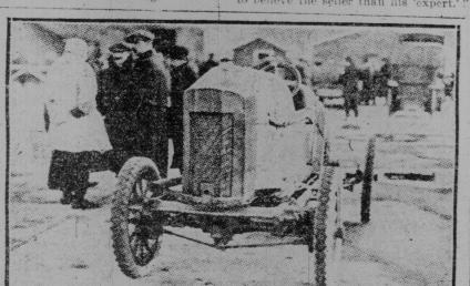
WHICH WAY DOES IT GO?-A RECENT WINNER AT BROOKLANDS. Curious radiator location on a 20.1 h.p. Brenna with "wind splitter" racing body. The radiator is placed at the rear and draft is induced the largest in the
