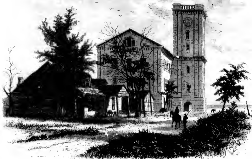
Old Arsenal, Rock Island.
