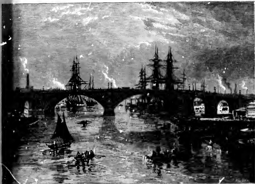
Chestnut-Street Bridge, on the Schuylkill.
