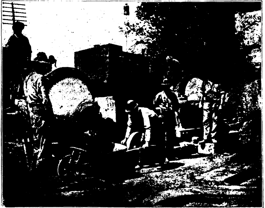
TWO SMITH MIXERS AT WORK ON CONCRETE BRIDGE AT ZANESVILLE, OHIO.
