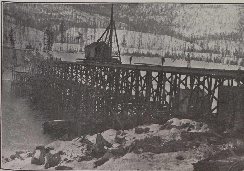
Fig. 1.—View Showing Falsework of the Bridge.
