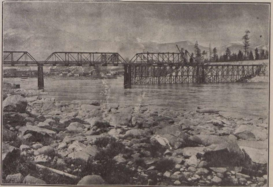
Fig. 2.—View Showing Falsework for Placing the Final Span.
