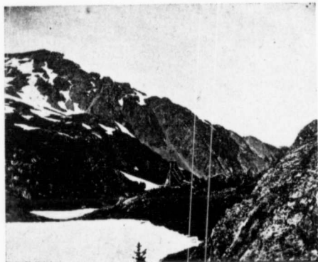
PTARMIGAN MINE, SHOWING GALLOWS FRAME.
