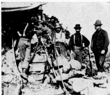
DIAMOND DRILLING ON THE PTARMIGAN MINE.
